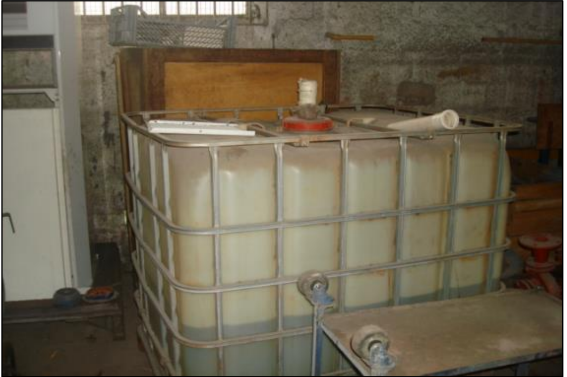
ITEM 5,345 - VISTA DO TANQUE GAIOLA 1000L
