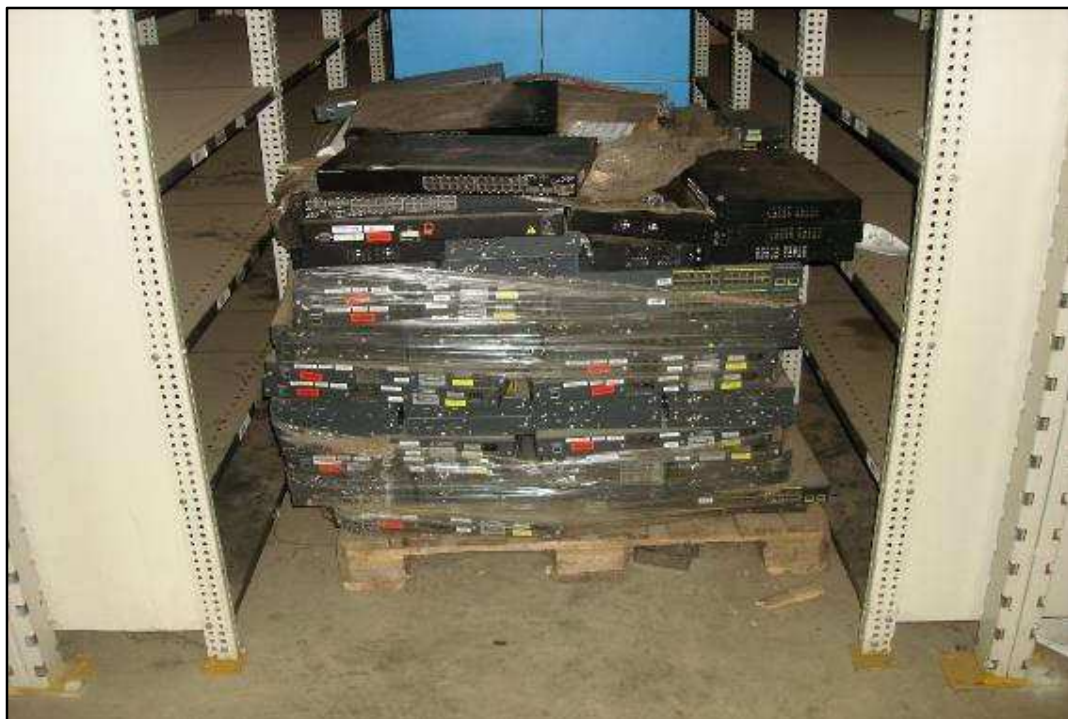
ITEM 2818 - VISTA DO DEL POWER CONECT 3524 E CATALYST 2960 MOD: 3524-2960
