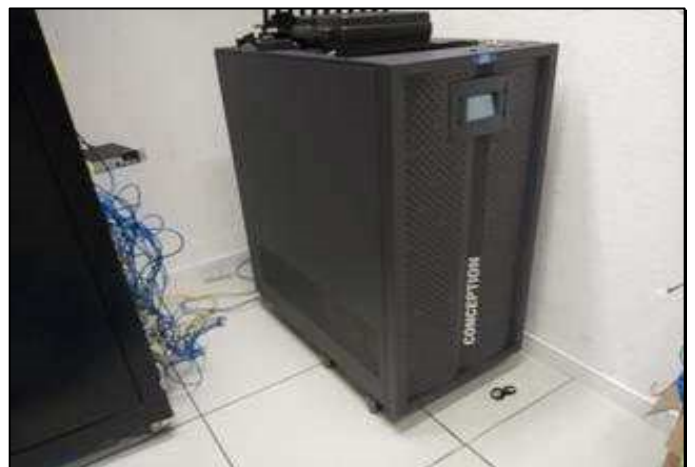
ITEM 1,439 - NOBREAK 30KVA CM COMMANDOS LINEARES CONCEPTION S1 LOCAL: SERVIDOR
