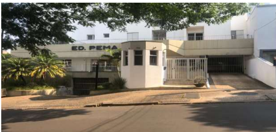
Portaria e acesso as garagens
