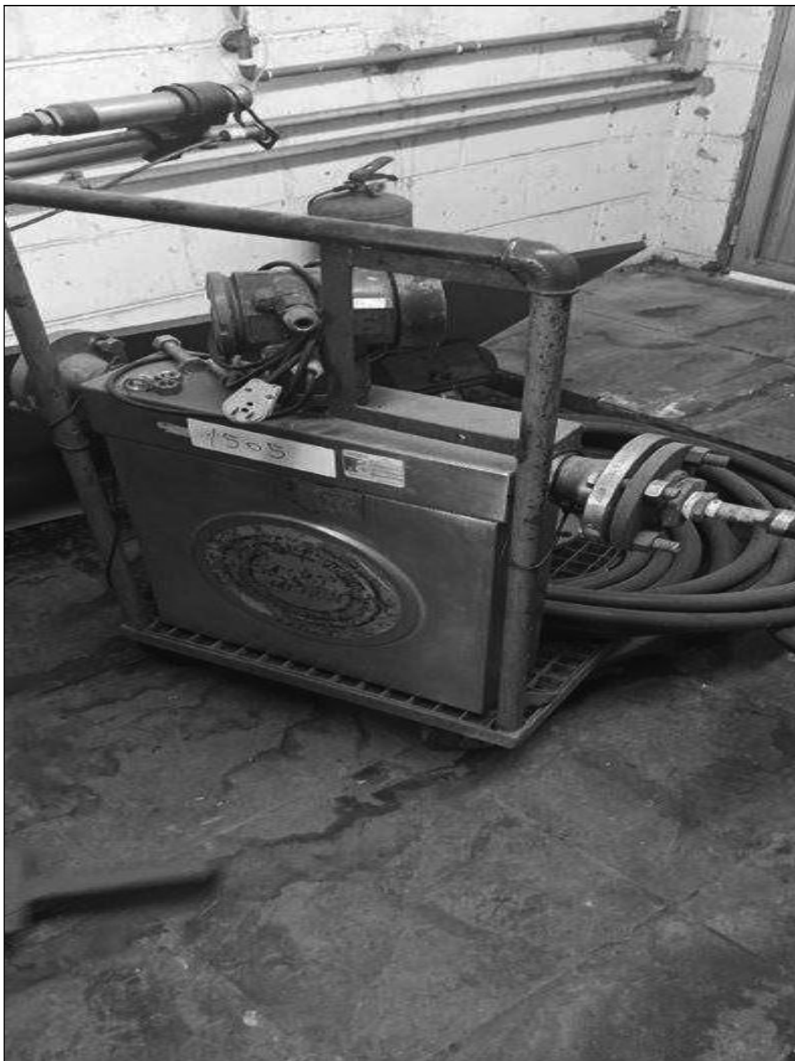
ITEM 1,001 – VISTA DO FT TRANSMISSOR DE FLUXO, FAB. MAICOLUX, MOD. F200S418SABZEZZZZ
