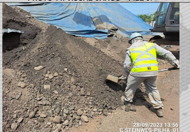
PHOTO 16: DURING INSPECTION – PILE 01
