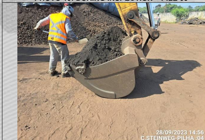
PHOTO 21: DURING INSPECTION – PILE 04
