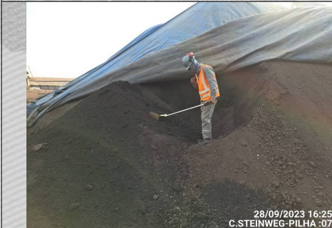
PHOTO 27: DURING INSPECTION – PILE 07
