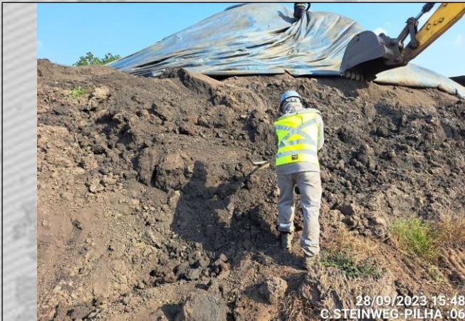
PHOTO 25: DURING INSPECTION – PILE 06
