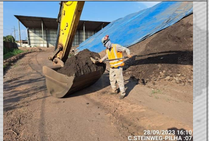
PHOTO 28: DURING INSPECTION – PILE 07
